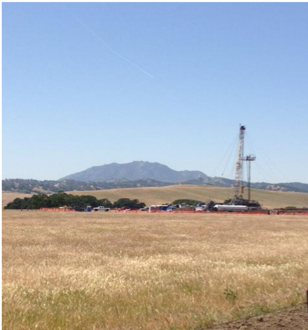
Graham Drilling Rig #4 looking West towards Mt Diablo
